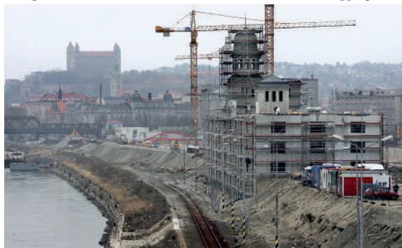
The construction of Eurovea was still on in 2007
