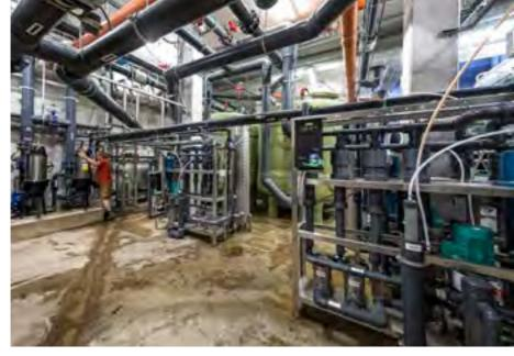
The area where the water for the hippo pools is cleaned resembles a little factory. It includes massive filters, ozonization and UV lamps. Altogether there is one kilometre of pipelines installed.
